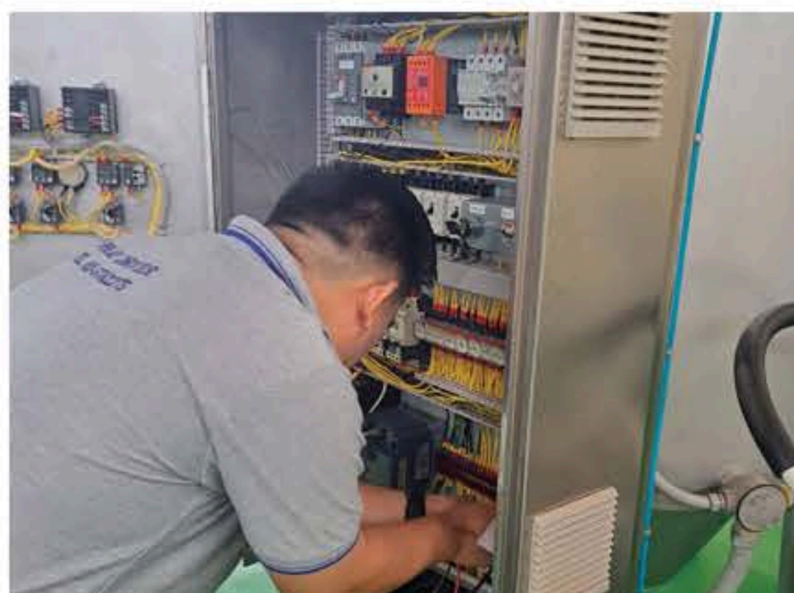
We provide maintenance and repair services for machinery at the Industrial Promotion Center Region 2, Department of Industrial Promotion (DIP), Phitsanulok Province.
