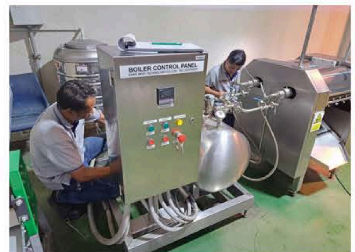
We provide maintenance and repair services for boilers and twin drum dryers at Mae Fah Luang University.
