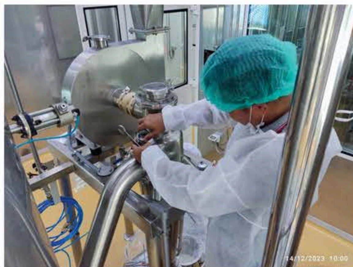
We provide maintenance and repair services for spray dryers at Suan Chitralada.
